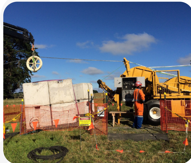
Figure 2: A full-size block should be used to avoid excessive bending around small guide rollers. Photo courtesy of Trans Power New Zealand.
