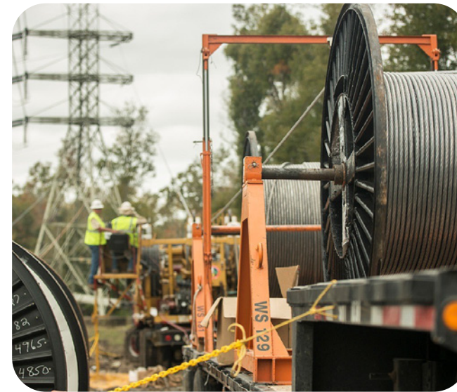
Figure 3: Pulling the conductor to ground to install the traveling ground is commonly done using a single rope. This could kink the conductor if tension was high enough. Use a 28x diameter guide roller, or slacken the conductor if it needs to be lowered to install the traveling ground. Photo courtesy of CenterPoint Energy.
