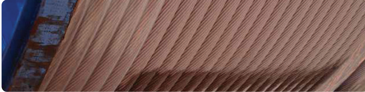
Figure 17: Water stain on conductor.
