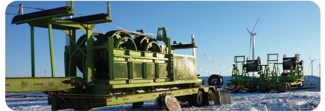
Figure 4: Payoff and bullwheel setup.
