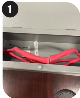
1 Identify the 2 cables to be spliced
